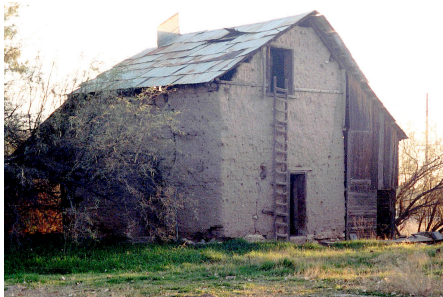
Pump house and blacksmith shop in 1990s
