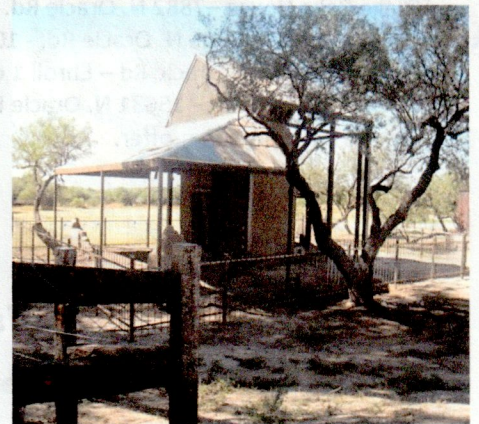
Steam Pump and Cover at Steam Pump Ranch
