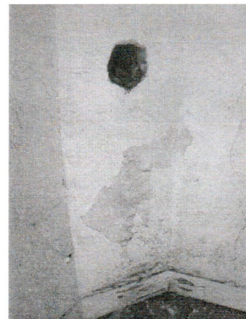
Remaining flue hole for wood burning stove in the livingroom.
