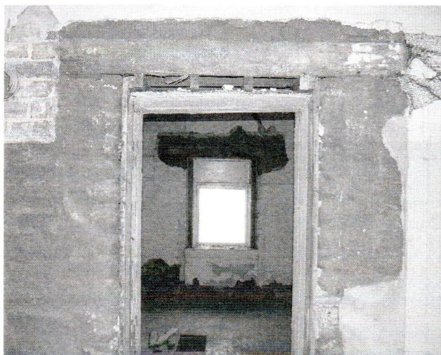
Exploratory removal of cement plaster reveals details of construction above kitchen door and bedroom window.
