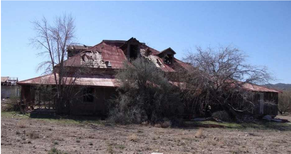
Feldman Ranch House - North End
