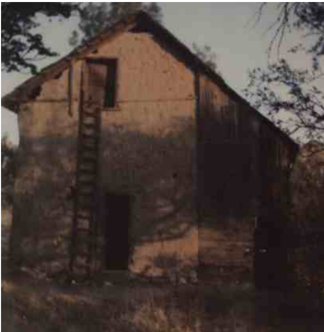
The West end of the adobe structure, looking east. The well and pump jack were located in the room just inside the door. The steam engine was outside the adobe structure on the right. There is a large window in the south side of the building to accommodate a large flat drive belt which connected the steam engine rotary output to the pump jack input drive wheel. See the last page for a sketch of the pump jack.
